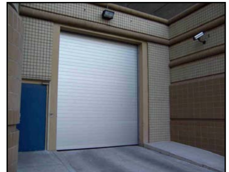
Clark County Detention Center
