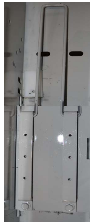
Fig 2. Safety brake deployed.
